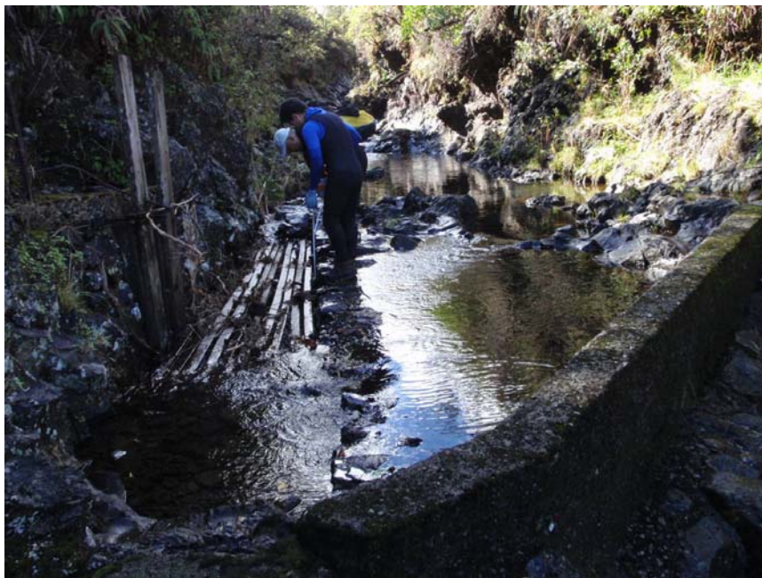
Figure 4-3. Concrete weir next to survey site 6. Photo is taken in the upstream direction. (2/11/2009; Tributary name: Kapā'ula (64021001); PBN: ts006p-123-021109; Surveyor: Shimoda, T.; Habitat type: Riffle; SBN: ts006n-021109; Lat. (DD): 20.80955, Long. (DD): -156.11530).
